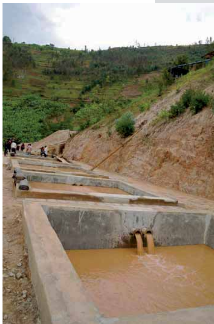
Effluent water settling ponds at Cyubi
