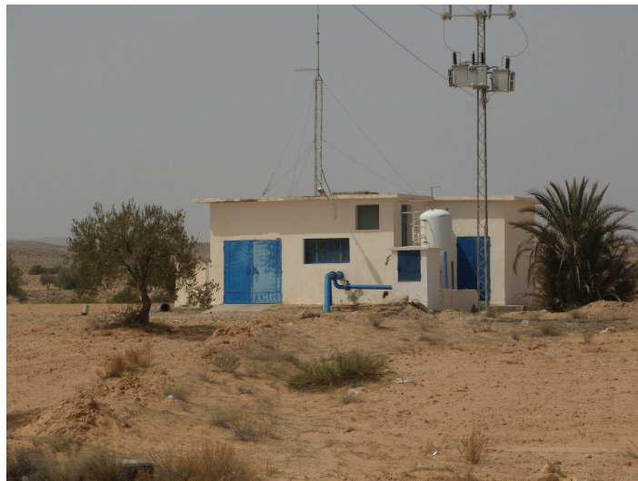
Photo 7. Pumping booster station.
