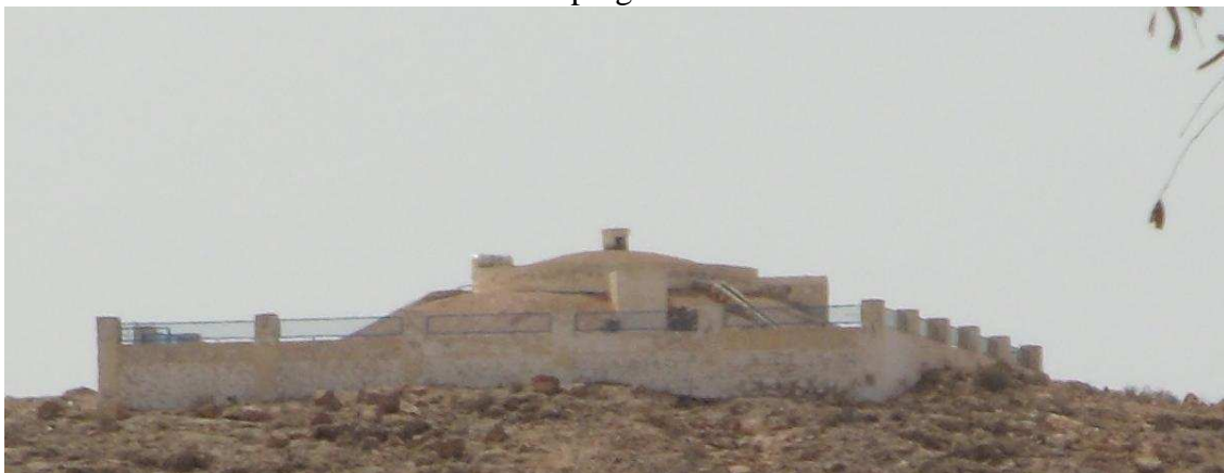
Photo 8. Example of drinking water tank.
