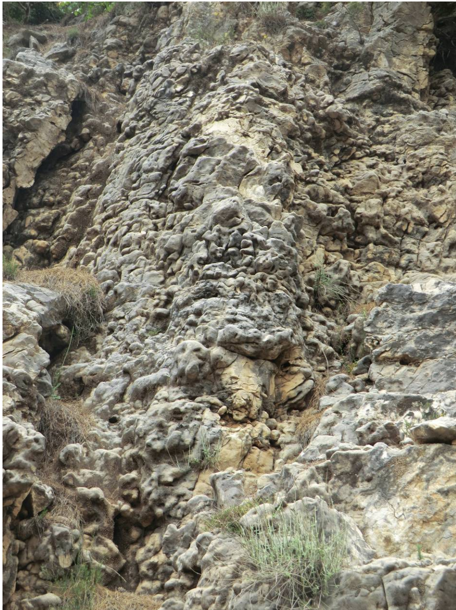
Photo 3: Secondary Dolomite near Planned Janneh Dam showing extensive Porosity
