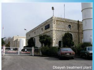
Dbayeh drinking water treatment plant was built in 1896. It's capacity is too small and it cannot treat inorganic constituents, heavy metals and other hazardous substances. The laboratory capacity is also insufficient to monitor pollution.
