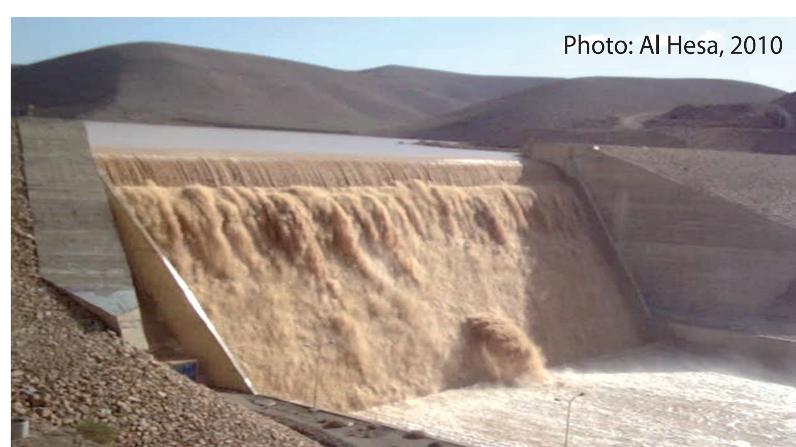
Figure 3: The mean annual inflow into the reservoir is around 10,4 MCM. From 2002-2011 around 73,9 MCM were stored, whereof 64,7 MCM recharged the aquifer and 6,7 MCM evaporated. A part of the inflow was lost by overflow events e.g. in 2010.
