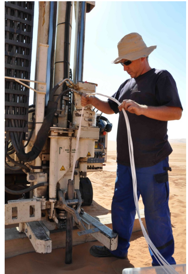
Installation of suction caps
