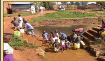
Figure 9. (A) Typical protected spring design (schematic); (B) Protected spring within the study area. Note the damaged spring protection wall and loss of drainage ditch, which contribute to direct entry of surface contaminants into the spring backfill during the rains
