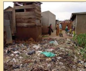
Figure 5. Typical raised pit latrine in the area. Note solid waste dump in the foreground
