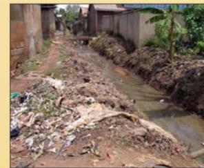
Figure 6. Sullage/storm water drain in the area with solid waste dumping on the drain bank.
