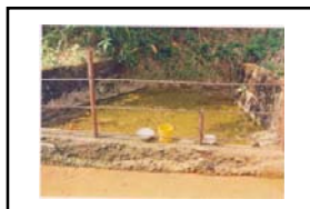
Poor environmental sanitation of shallow groundwater supply sources
