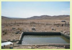
Picture 1: Infiltration basin and observation wells [Zemann, 2008]
