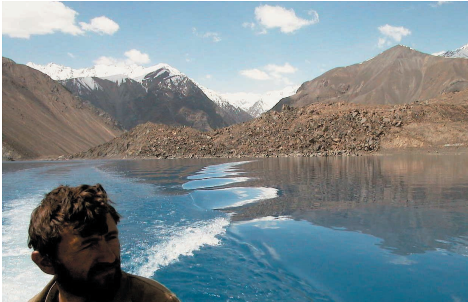
South end of the Usoi dam, showing the mixture of fine-grained and very coarse-grained angular material.
