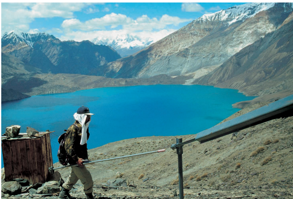
Lake Sarez from the mountain slope on the north side looking towards the dam; the landslide source area can be seen on the right side of the dam. The extensometers installed to monitor movement of the slope are visible in the foreground.
