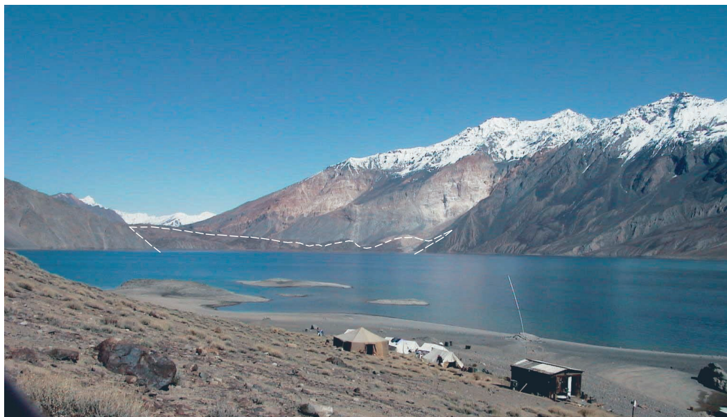
Lake Sarez (elev. 3260 m) and the camp of the monitoring team; the landslide dam is seen in the background (marked by the dashed line); the source area of the landslide can be seen to the right of the dam.
