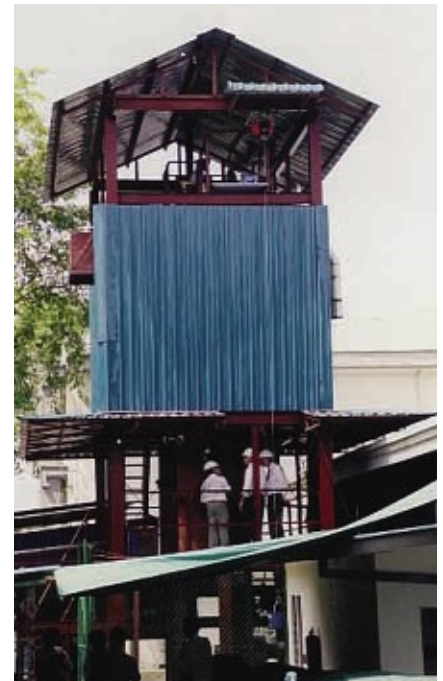
Demonstrationsanlage in Kuching, Sarawak, Malaysia.
