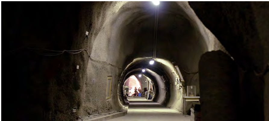
Stabilisation (shotcrete and lining) in a mining gallery in claystone
