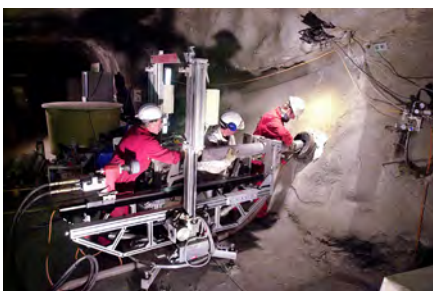
Stress measurements in rock with BGR's overcoring probe
