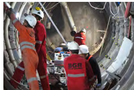
In situ geophysical measurements conducted from a tunnel wall
