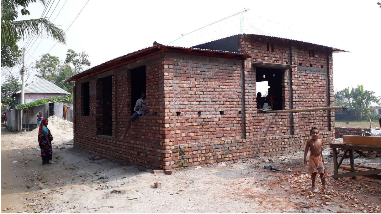
Figure 24: Residential neighbourhood adjacent to brick factories is showing strong subsidence.
