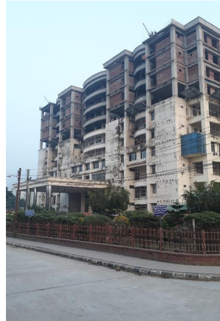
Figure 20: Construction in progress on the Faridpur Medical College campus.
