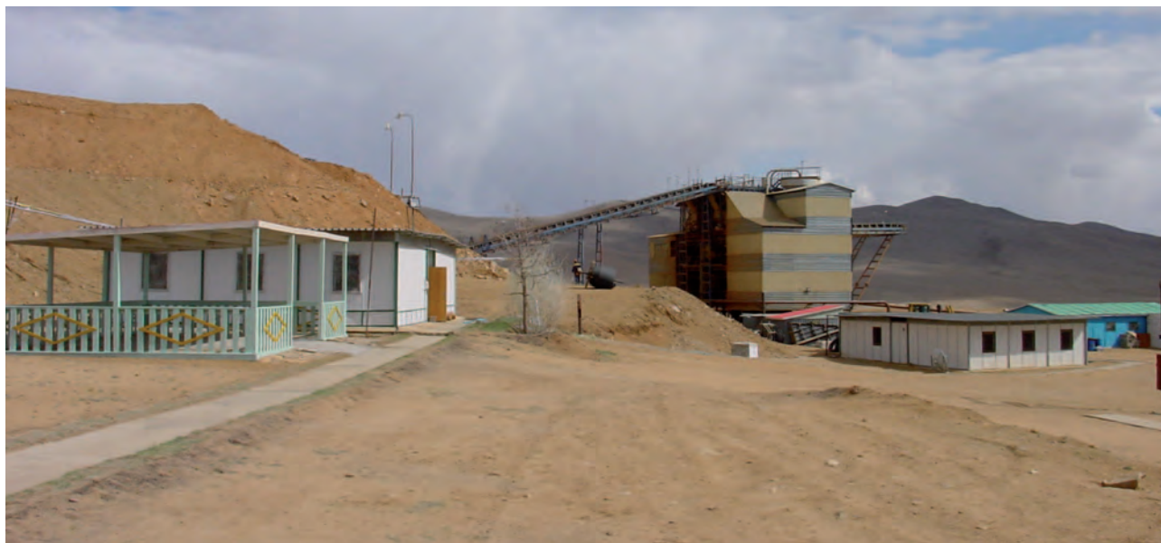
Figure 117: Beneficiation plant of NATIONAL MONGOLIAN COMPANY, East Khujkhaan.
