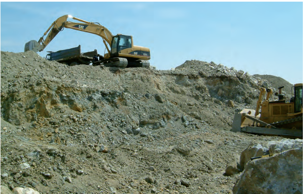
Figure 49: Mining at Chuluut Tsagaan Del on behalf of MONGOLCZECHMETAL LLC in May 2008.
