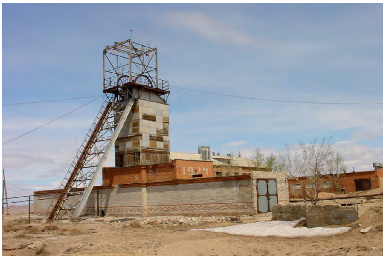
Figure 38: Former shaft of the Berkh fluorite mine as of June 2008.
