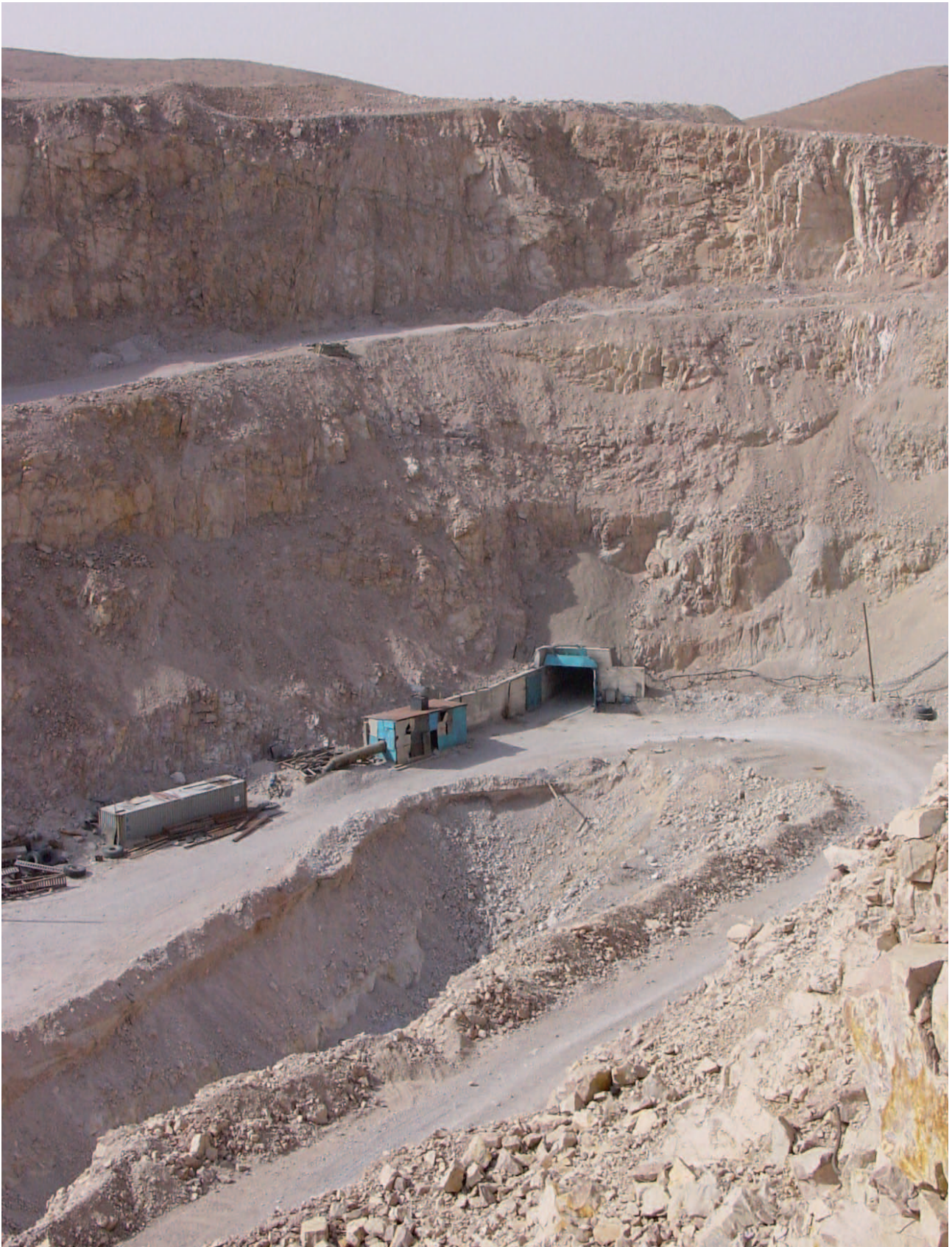
Figure 21: Former Adag open pit as of May 2008. Ventilation adit of the more recent underground mine in the middle of the photo.
