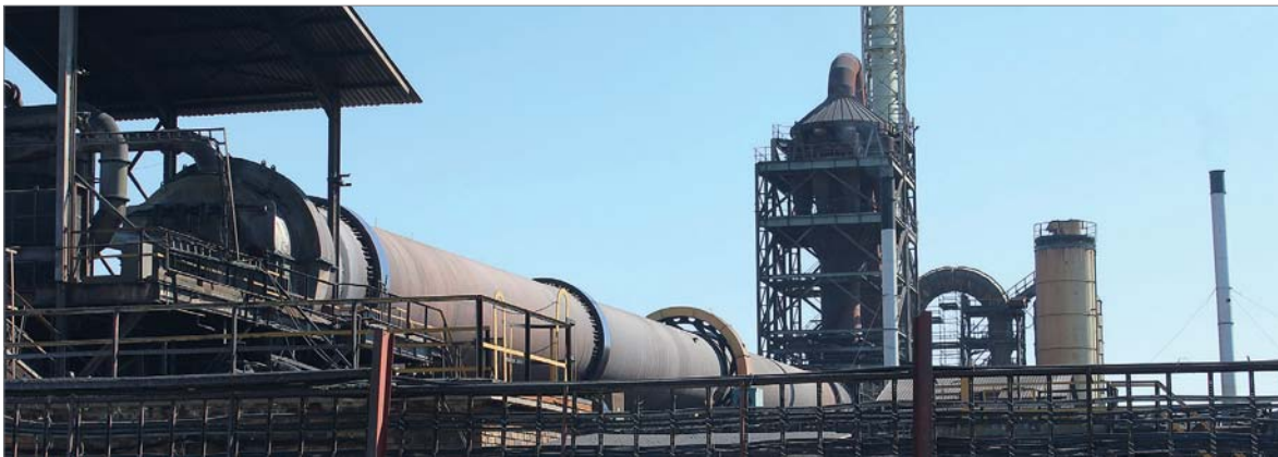
Fig. 3.14: Rotary kiln to produce vanadium pentoxide at the Rhovan plant (photo: DERA 2015).
