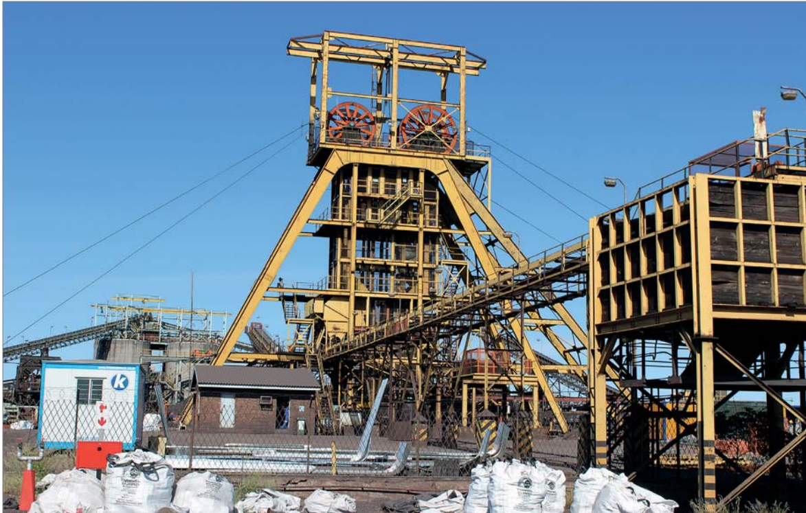
Fig. 2.11: Winding shaft at Hotazel mining area (photo: DERA 2015).
