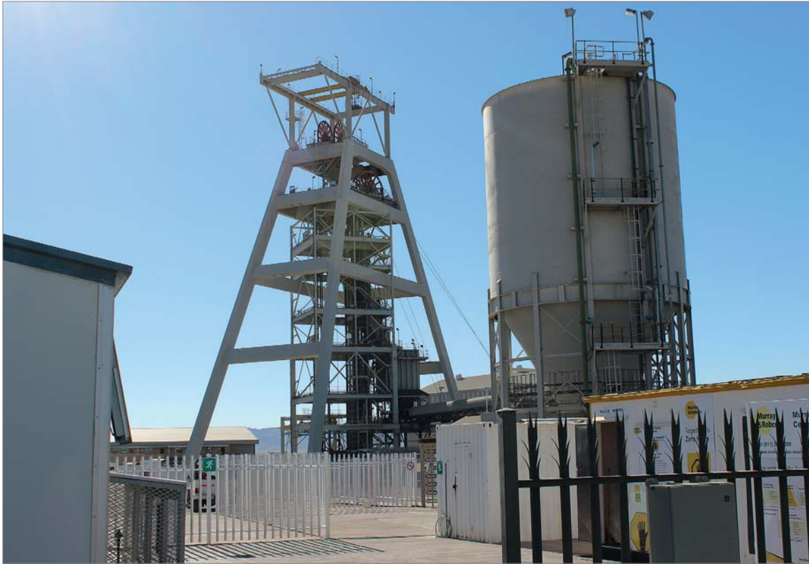
Fig. 4.6: Head frame of the “Deeps” shaft at Black Mountain (photo: DERA 2015).
