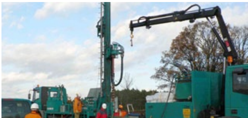
Installation of CO 2 monitoring wells.
