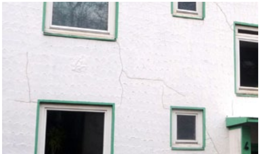
Residential area in Bremerhaven: cracks and tilted buildings as a result of insufficient foundations in the marsh sediments.
