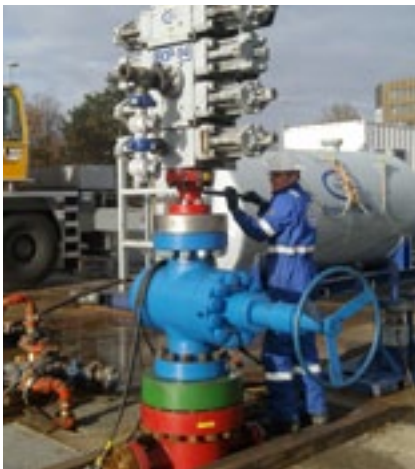
Wellhead being prepared to flush the well clean.
