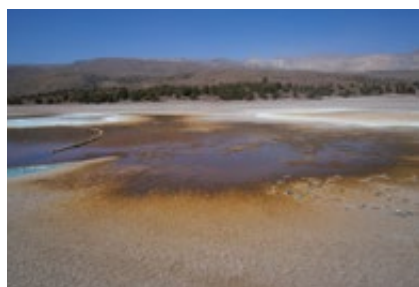
▲ Precipitation of mobilisates on the top of a tailings impoundment: iron hydroxide (reddish) and copper sulphate (blue, white).
