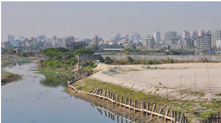
▲ New building plots are created at the edge of the capital city of Dhaka by filling in areas with sand.
