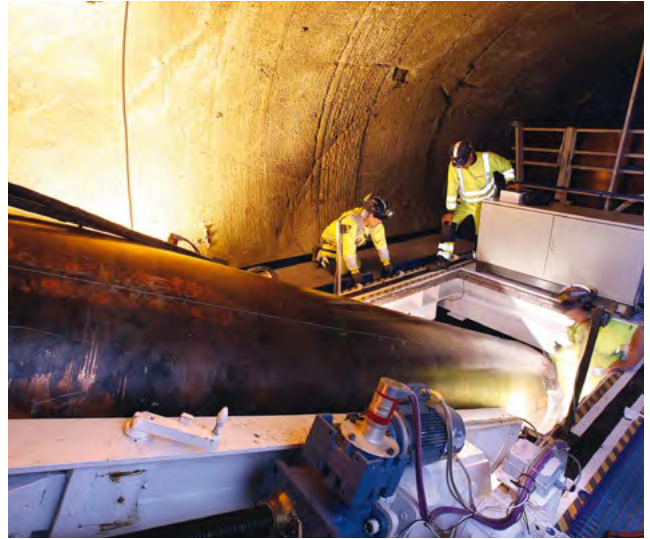
▲ Employees of the Swedish company SKB install the dummy containers for the radioactive waste emplacement test in underground test tunnels in the Swedish Äspö Hard Rock Laboratory.
