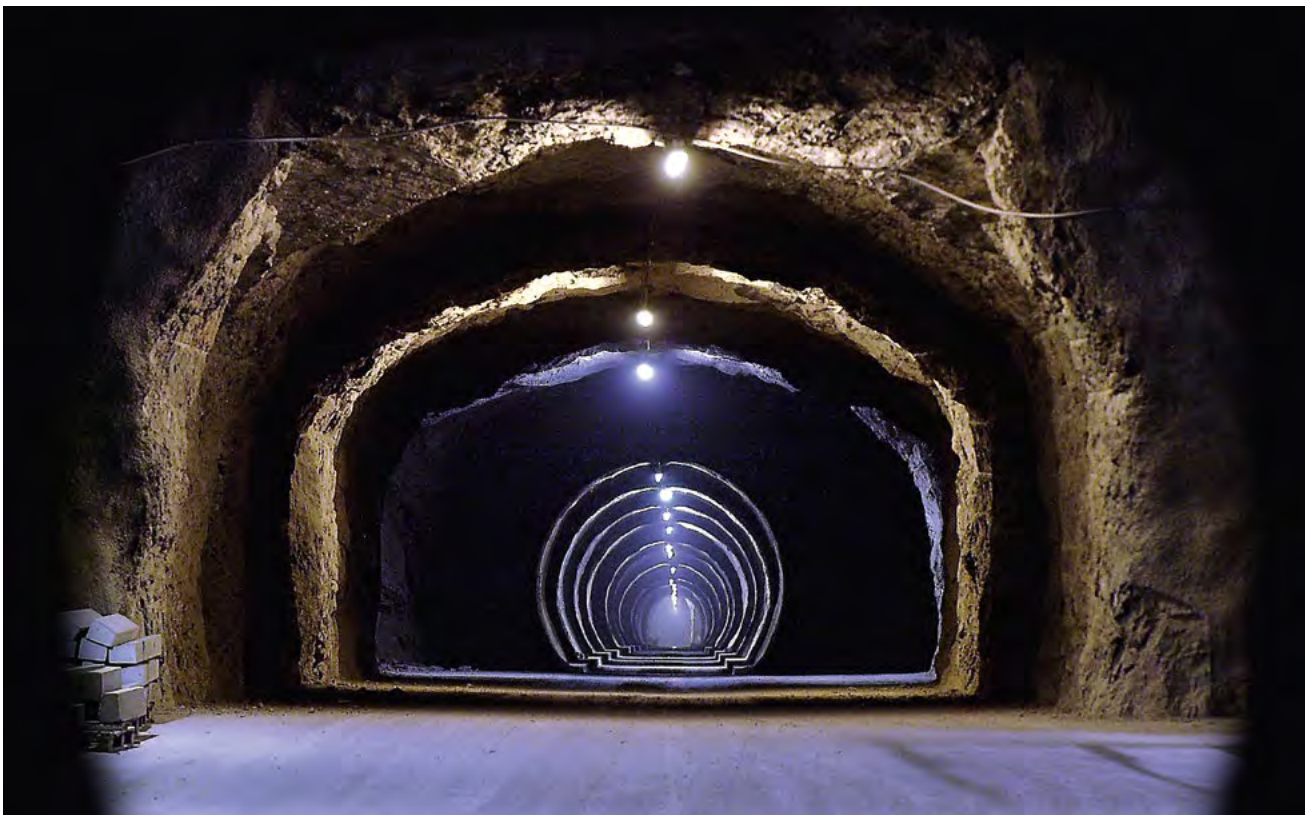
▲ Gallery in the international Mont Terri Rock Laboratory in Switzerland. BGR has been doing research here for 20 years, investigating the properties of claystones as a host rock for a repository.
