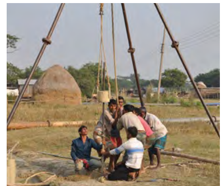
▲ Exploratory drilling to analyse the subsurface conditions.
