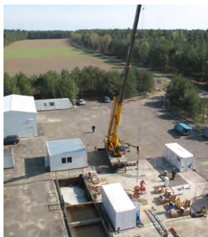
▲ Horstberg drilling site during the installation of a production pump.
