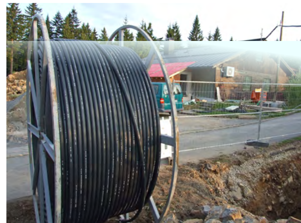
GERES facility on Sulzberg: All the GERES array seismometer monitoring points are connected via cable to the central power supply and data acquisition in this building.
