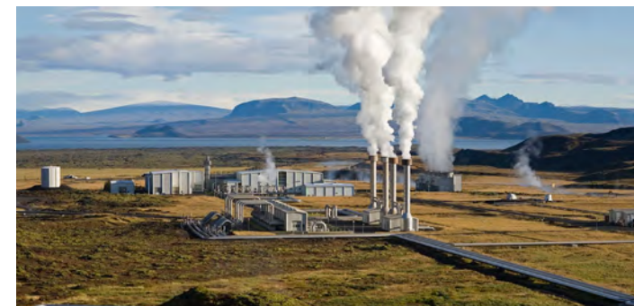
Icelandic geothermal power station.
