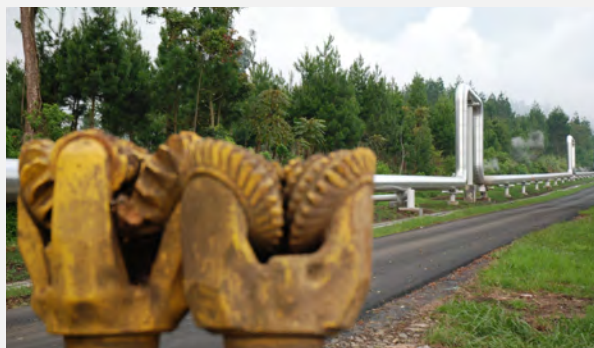
Pipelines at the 200 MW Kamojang Geothermal Power Station, West Java.
