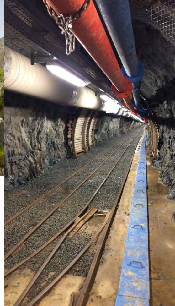
Underground laboratory in crystalline rock.
