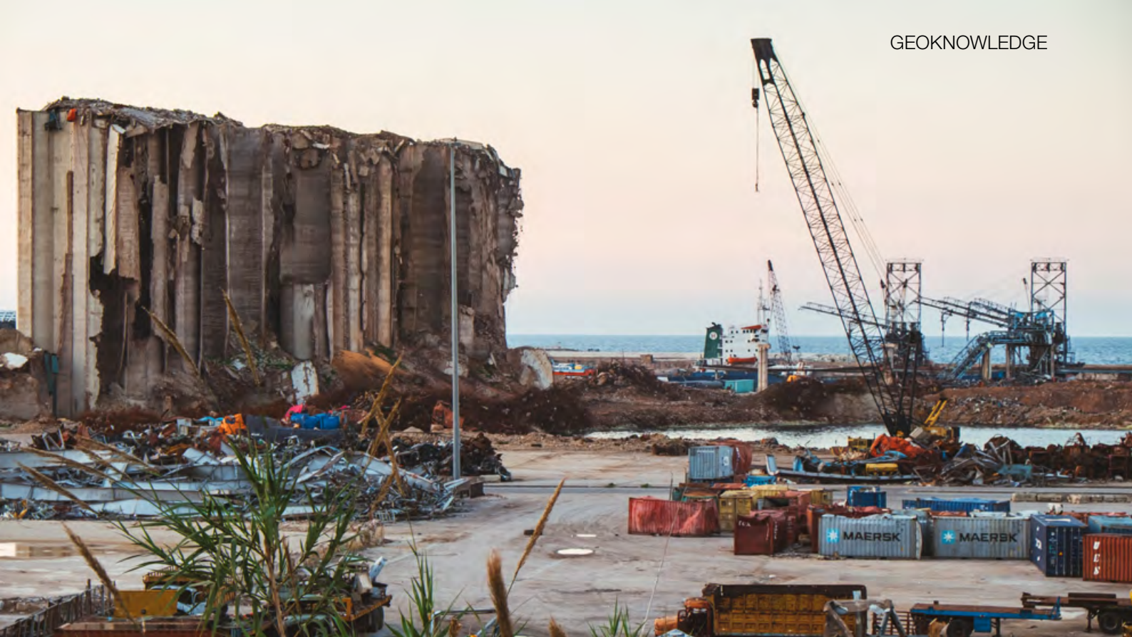
The blast in the Port of Beirut caused severe destruction to buildings and infrastructure within a radius of several kilometres around the explosion site.
