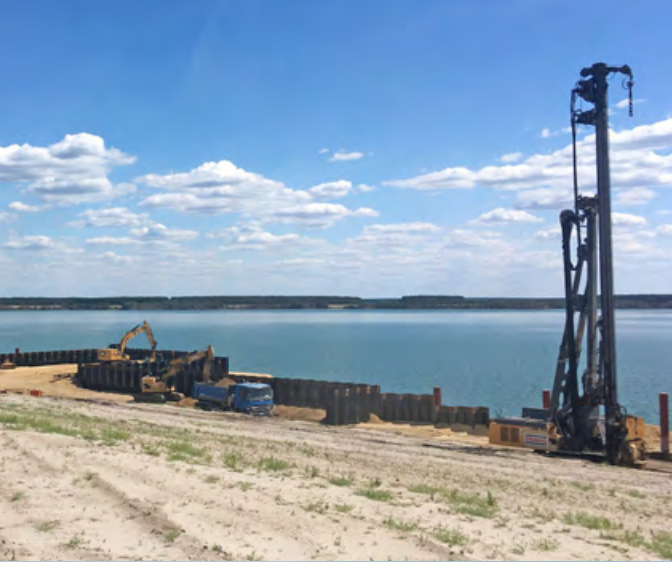
Measures to stabilise the shoreline of an artificial lake as part of the rehabilitation of a decommissioned open-cast mine.
