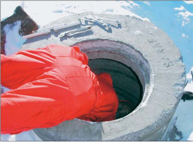
Work being carried out at station AS035 during the certification test.
