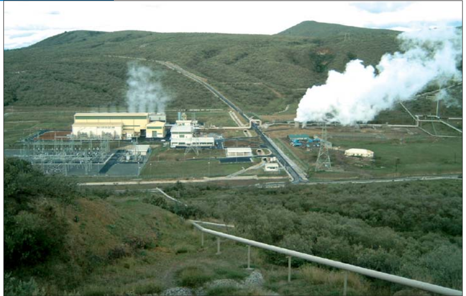
Geothermal steam power plant at Olkaria II, Kenya, with approx. 70 MW electrical output.
