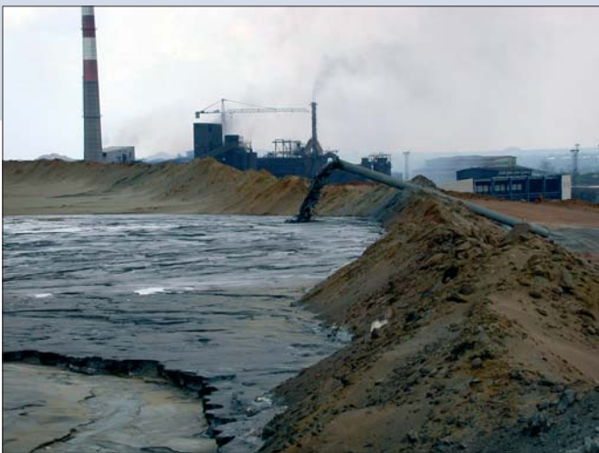
Dumping processing residues on a mine tip. The ore treatment plant is shown in the background.
