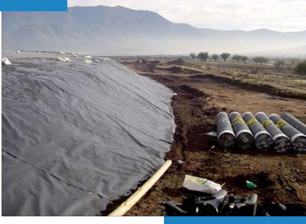
The project training programme included the preparation and implementation of pilot clean-up activities right at the start of the first phase, as shown here with the containment of a land-fill which contains toxic residues from the processing of gold ore.
