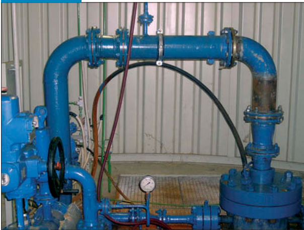
Well head installation of the Neustadt-Glewe production well.
