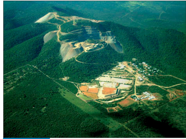
Aerial view of the Okorusu fluorspar mine in the highlands of northern Namibia.
