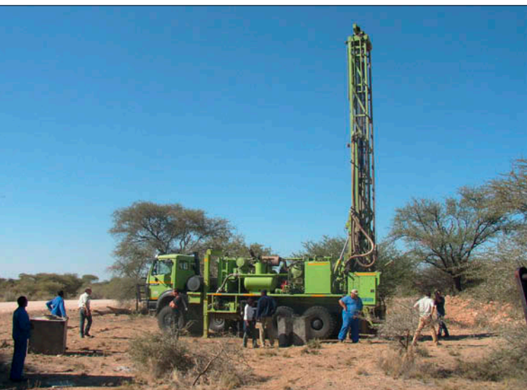
DWA drilling crew at work in Caprivi.
