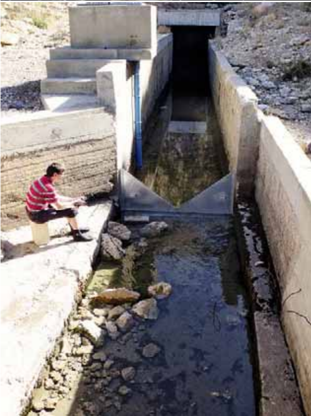
(above right) Spring capture at the Figeih spring (Syria) at its outflow from the rock.
