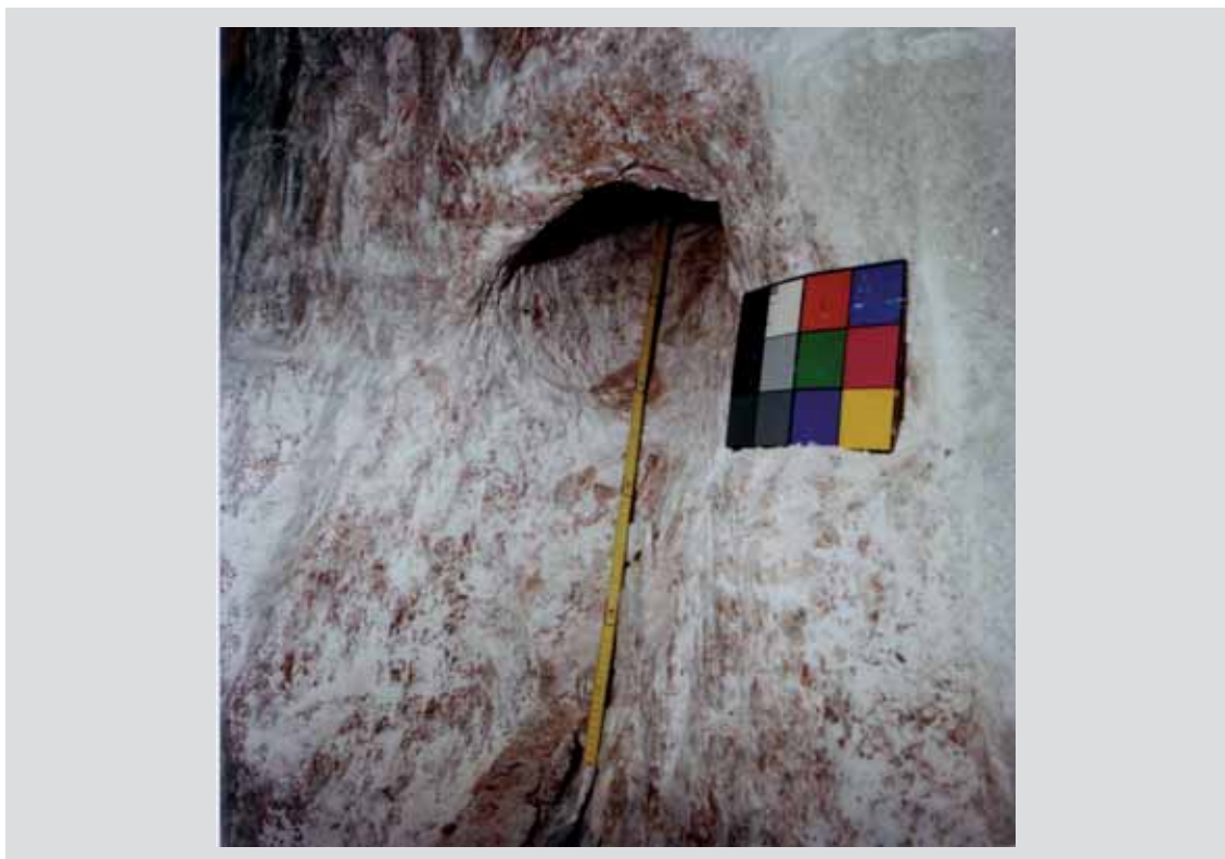
Figure 48: Gas flute in the Kaliflöz Stassfurt. It was formed when excavation work in the potash seam caused the release of gas that had been embedded under pressure in the brecciated carnallite (crackling carnallite). The flute is approx. 1.5 m long and has a diameter of approx. 30 cm. Cross-cut 1 West, 840 m-level, drift position 85 m, western wall. (Photograph: Bauer, DBE)
