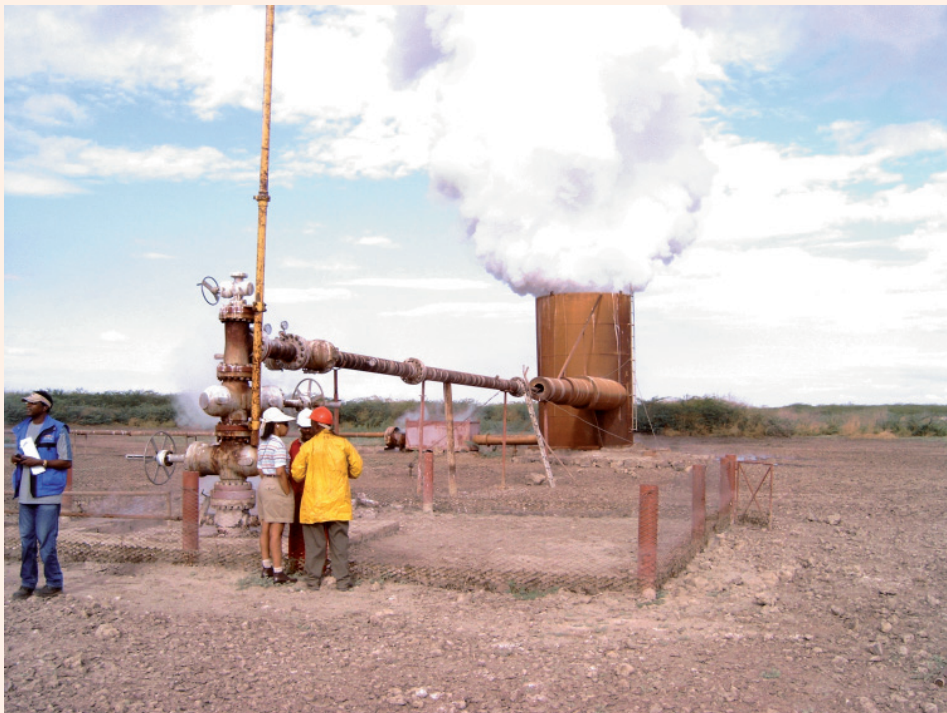
Production at an exploration well in the geothermal field Tendaho, Ethiopia
