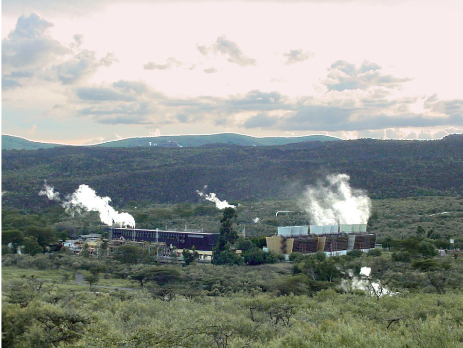
Figure 7.9: The geothermal power plant Olkaria I in Kenya started generating power from geothermal energy in 1981. Currently 45 MWe have been installed; the average availability is more than 98%.
