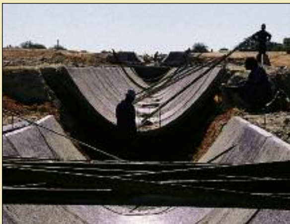
Grootfontein-Omatako Canal under construction
