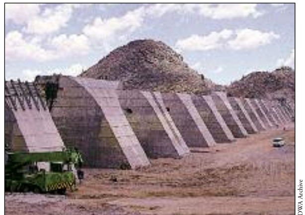
The Otjivero Dam main wall under construction
