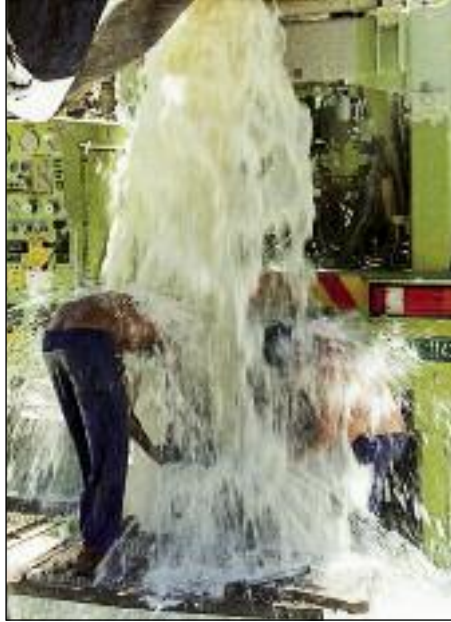
Under pressure! Borehole penetrating the Oshivelo Artesian Aquifer with a free flowing yield of more than 200 m 3 /h.
