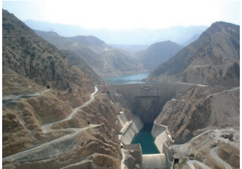
The Karun-3 Dam on the Karun River, Iran, 2008. Source: M. Samadi.
