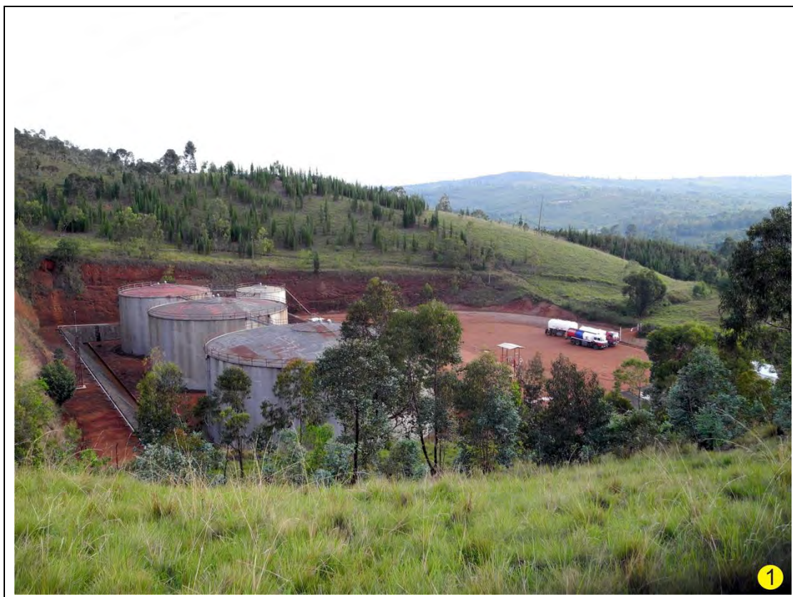
Figure 7.2: View to SE onto a petrol storage. Leakage could possibly cause contamination through open faults at wells downstream.
