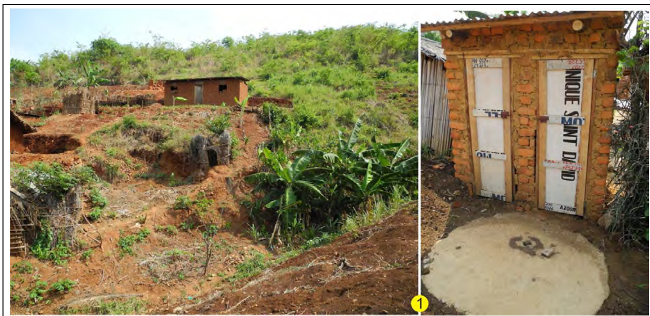
Figure 7.7: View to NE (WP 83). Pit latrines in this fault may cause water contamination. Right: sealed toilets nearby are a good step towards a better solution.
