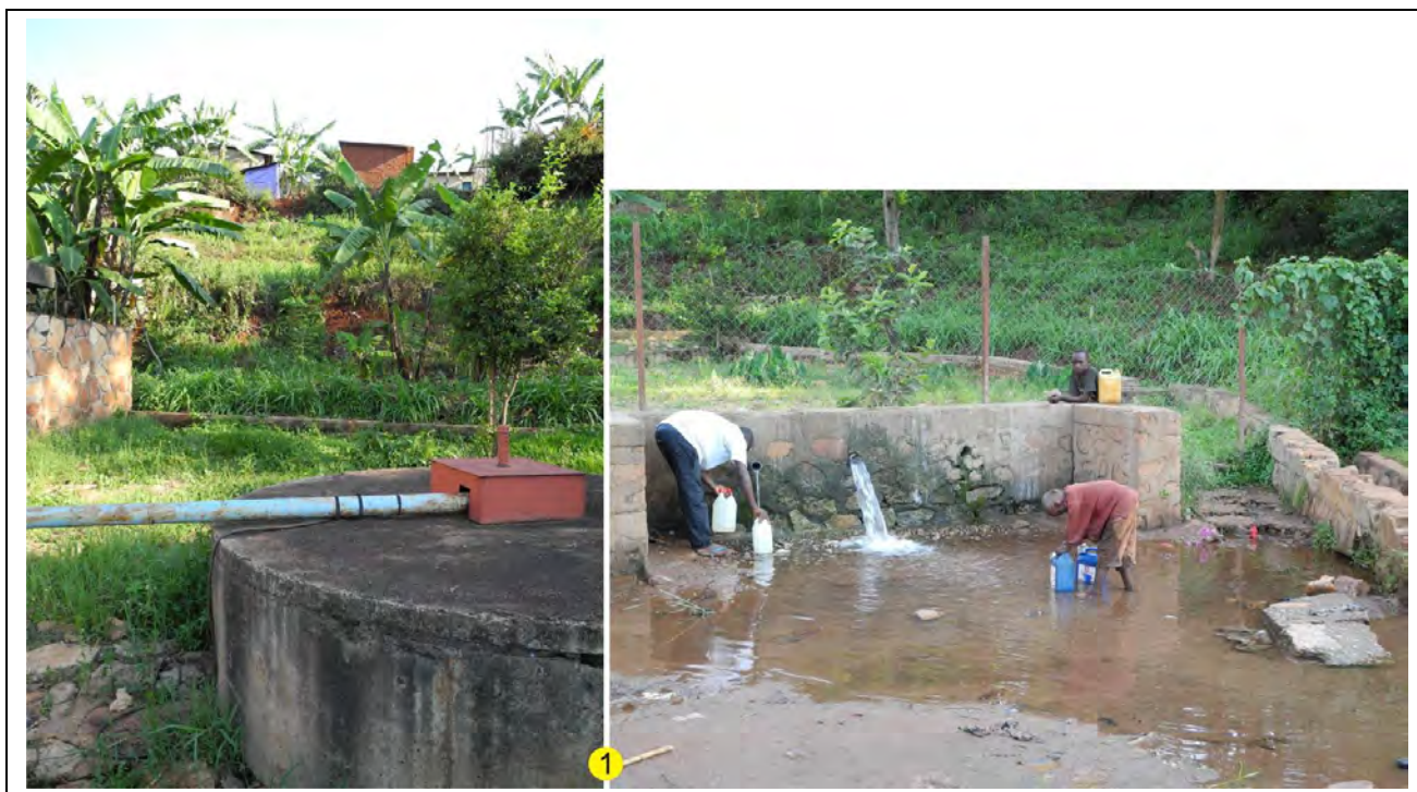
Figure 7.5: View to the south (WP 11). High bacteria content of these wells at this pump station may be caused by pit latrines directly uphill. The pond directly to the right functions also as a car wash. A small slaughterhouse nearby may cause further contamination.
