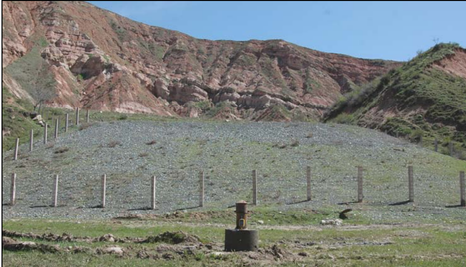
Figure 5. Tailings impoundment no. 3 with a newly constructed groundwater-monitoring-well in the front.
