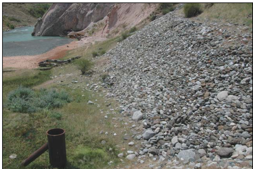
Figure 16: Continuous discharge of seepage water (Station 11) of tailings impoundment no. 5.
