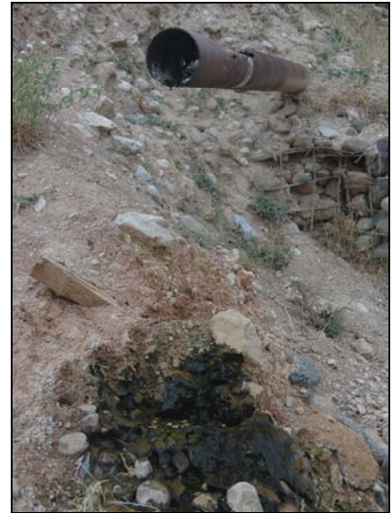
Figure 17: Outflow of seepage water (Station 14) at the bottom of tailing no. 16.
