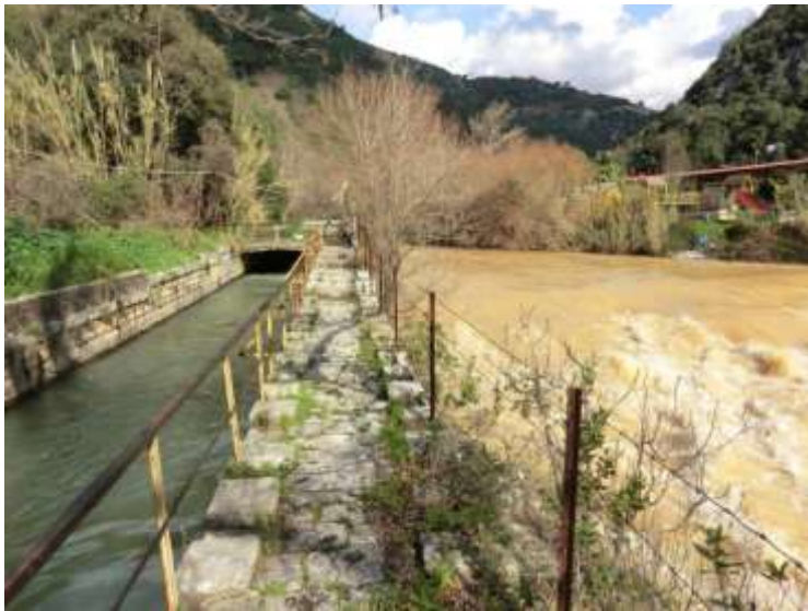
Figure 4-47 Mokhada Diversion Station during Wet Season (26-01-2012)
