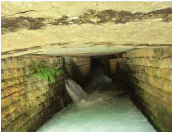
Figure 4-40 Inside of Canal at Mokhada Diversion Station
