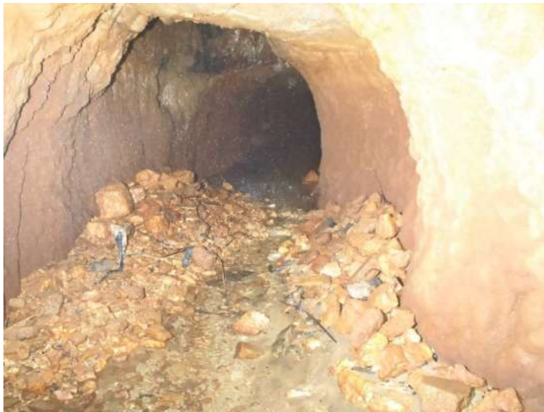
Figure 4-61 Rock Falls in Tunnel (picture: BMLWWE)
