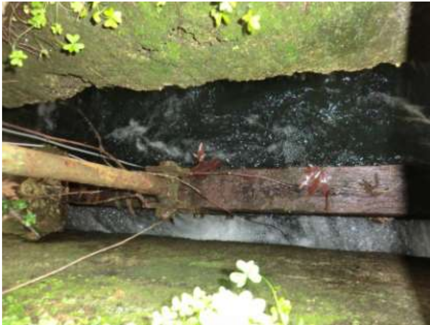
Figure 4-69 Dysfunctional Weir
