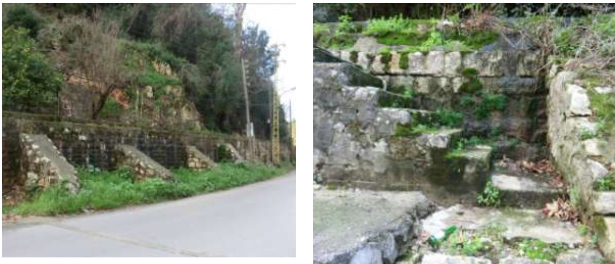
Figure 4-74 Diverse Leakages from Canal (Leakage-2 and Leakage-3)
