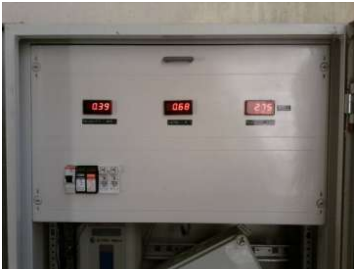
Figure 4-37 Measurement of Flow Velocity/Water Level at Kashkoush Spring
