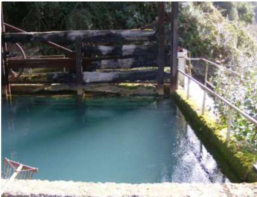
Figure 4-28 Diversion Dam (Component 5)
