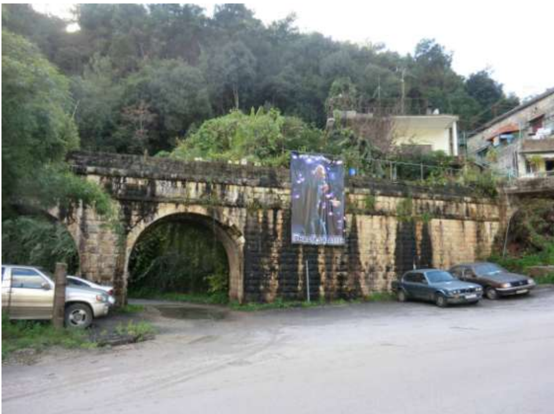
Figure 4-76 Location of Leakage-4
