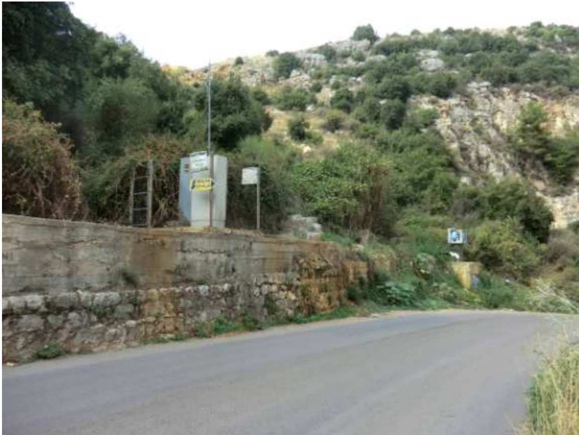
Figure 4-59 Nahr el Kalb-Dbaye Tunnel
