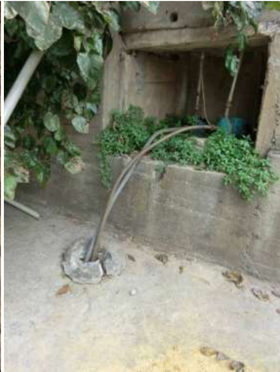
Figure 4-54 Households tapping into the Jeita-Dbaye Canal
