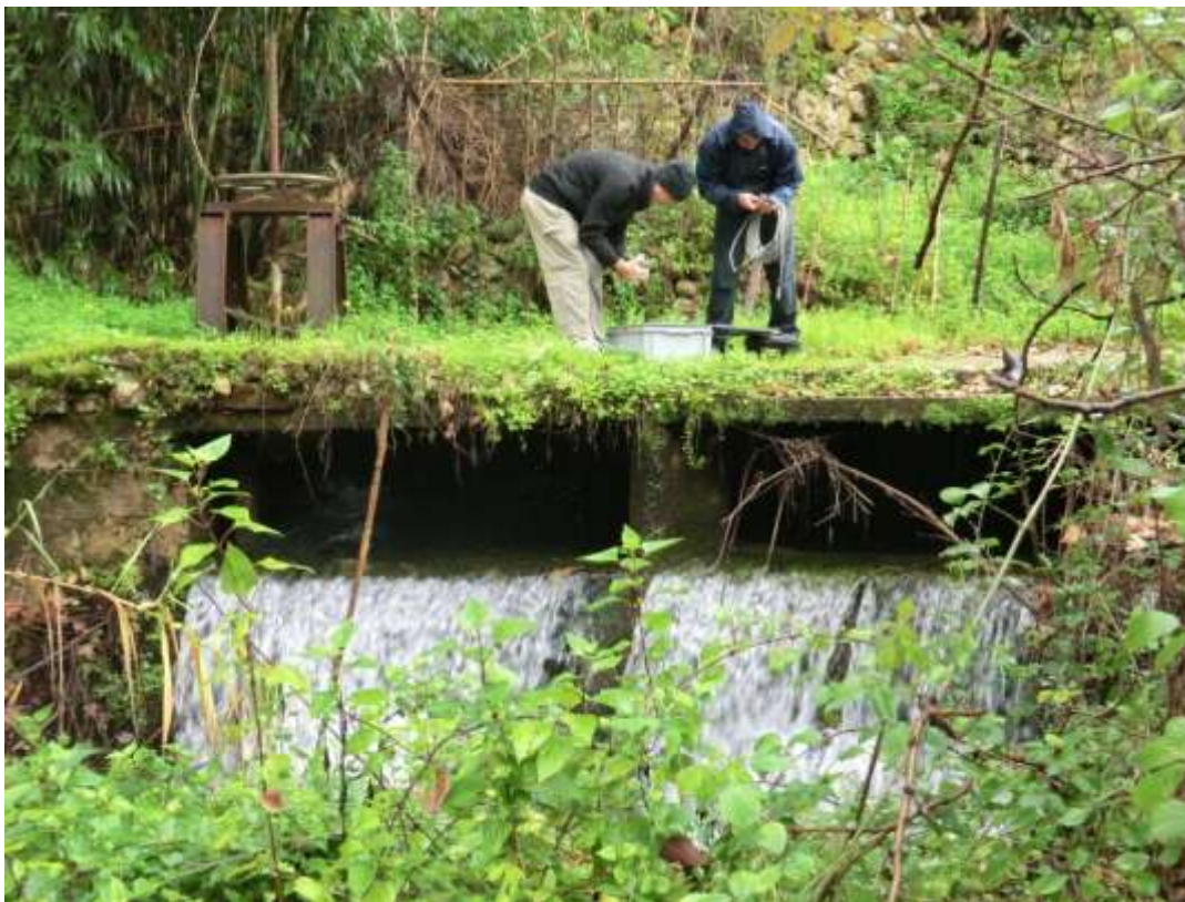
Figure 4-68 Overflow due to Dysfunctional Weir
