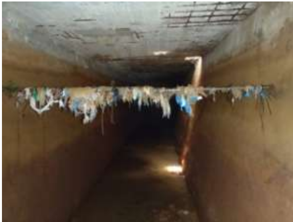
Debris from the OEB Dam intake
