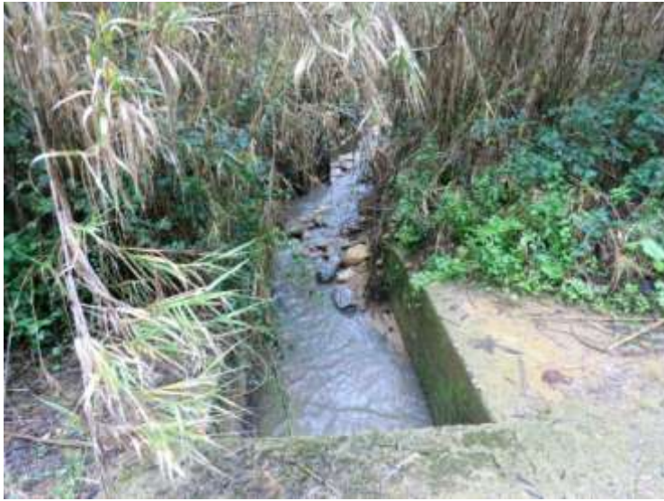
Figure 4-44 Wastewater overpass of Jeita-Dbaye Canal
