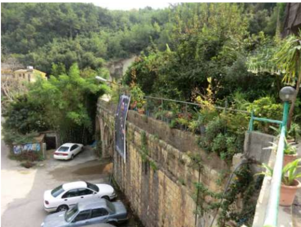
Figure 4-58 Canal used as a Garden in Mokhada near Aqueduct
