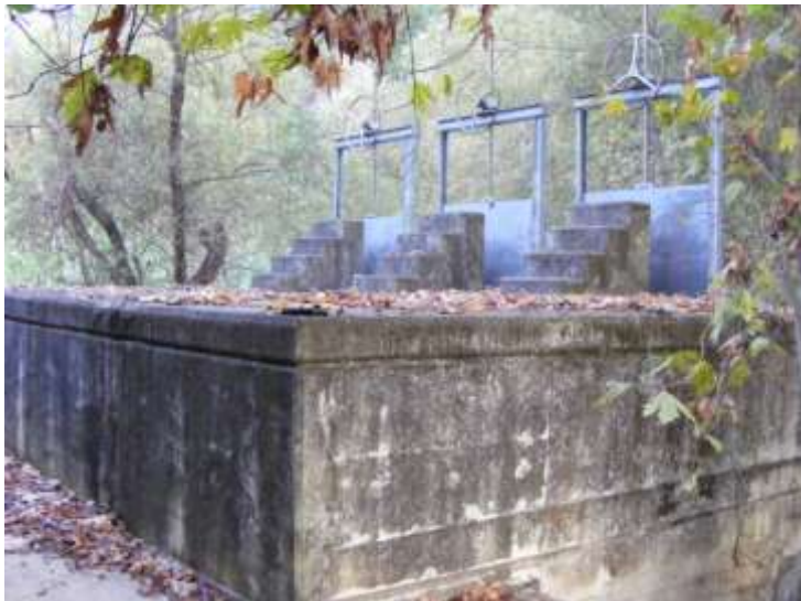
Figure 4-38 Kashkoush Spring Intake downstream of Harch HPP
