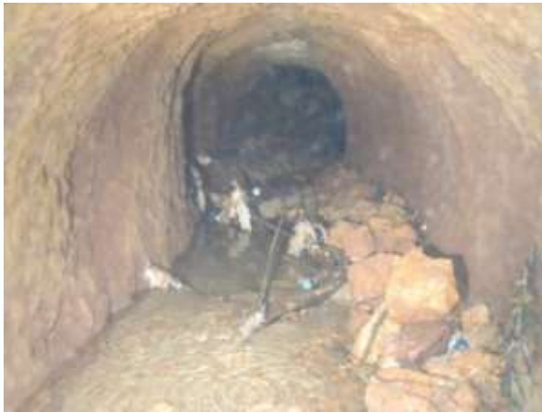
Debris in the channel
