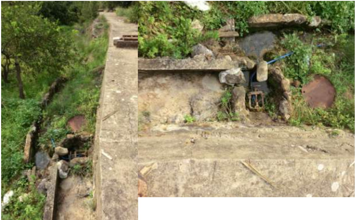
Figure 4-46 Irrigation Water drawn from the Canal
