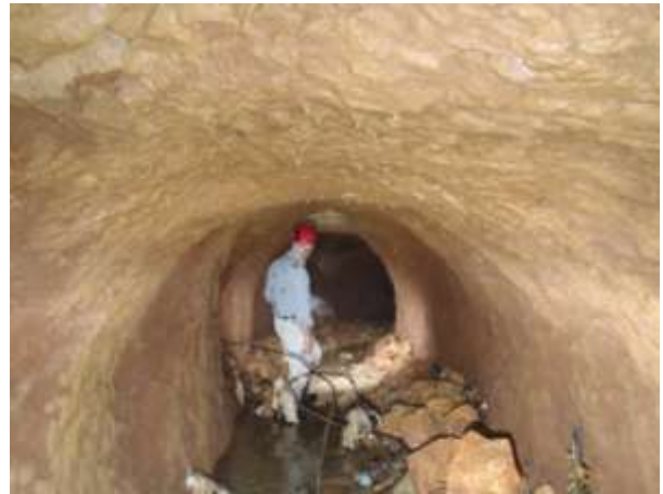
Debris in the channel
