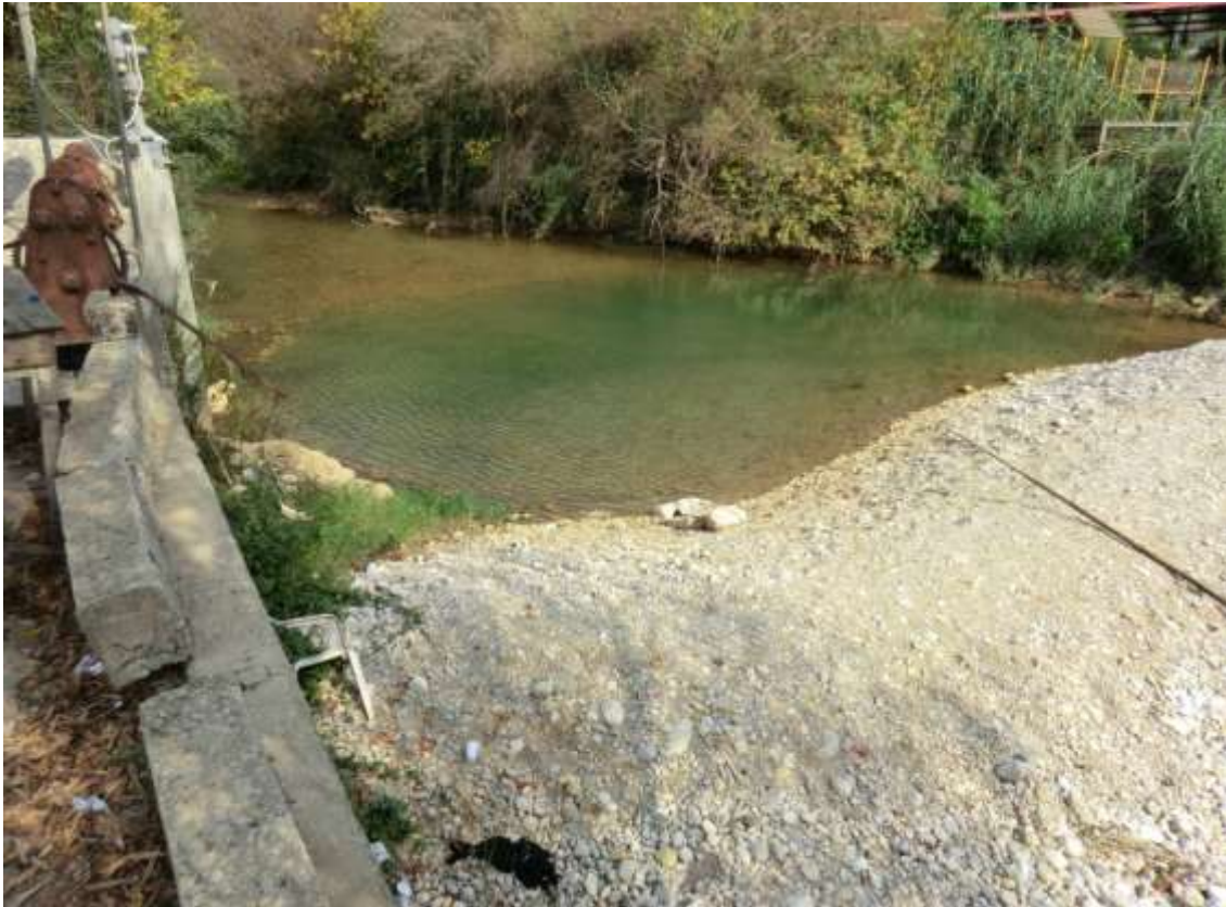
Figure 4-52 Summer Water Intake at Mokhada "Dam" (Diverting Water from Nahr el Kalb into the Canal during summer time)
