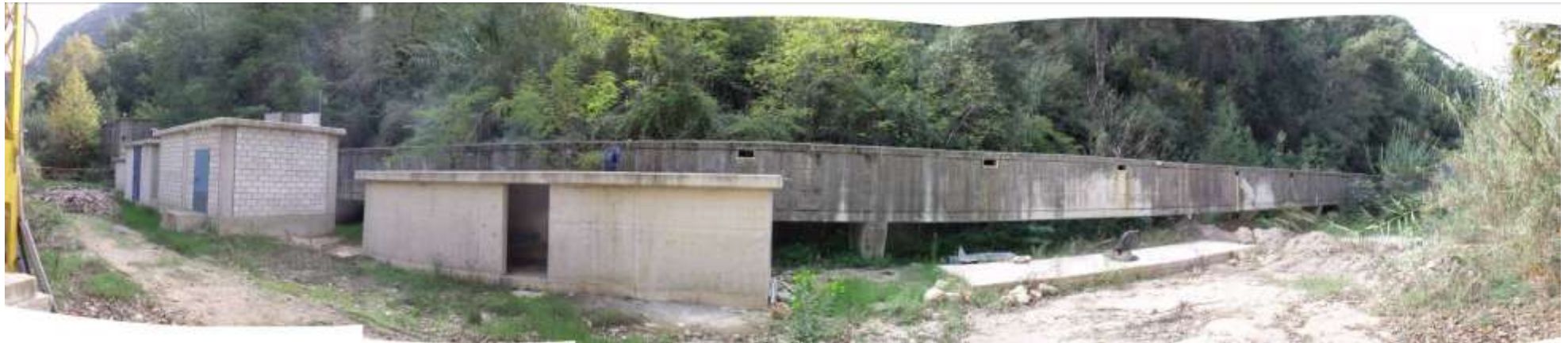
Figure 4-30 Kashkoush Well field and Outlet of Kashkoush Spring
