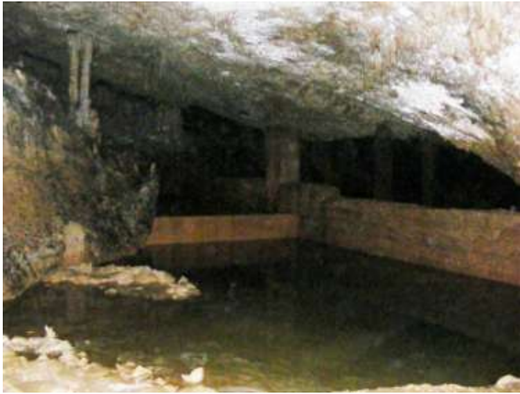
Figure 4-6 Inner Dam with Intake to Tunnel
