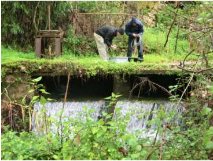
Figure 4-41 Overflow due to Dysfunctional Gate near Mar Abda Bridge
