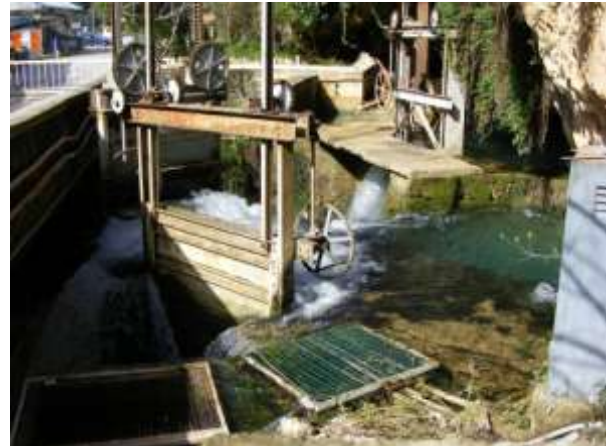
Figure 4-10 Overflow from Outer Dam
