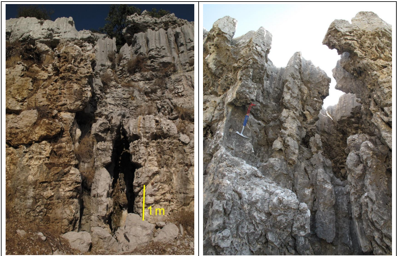
Figure 67: Left: Entrance to sinkhole further pathway blocked by fallen rocks after approximately 10 m (WP 229). Right: Deeply (> 10 m) karstified J4, 1.5 km SE Marjaba (WP 032)
