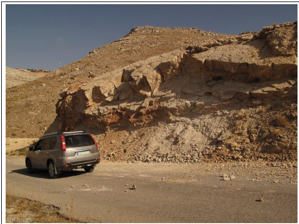
Figure 63: Rock fall consisting of huge blocks of mainly C4-limestone. Blocks are dipping with slope, endangering roads and new-built houses inside this area of a housing estate 1 km south east of Faqra (WP 263)
