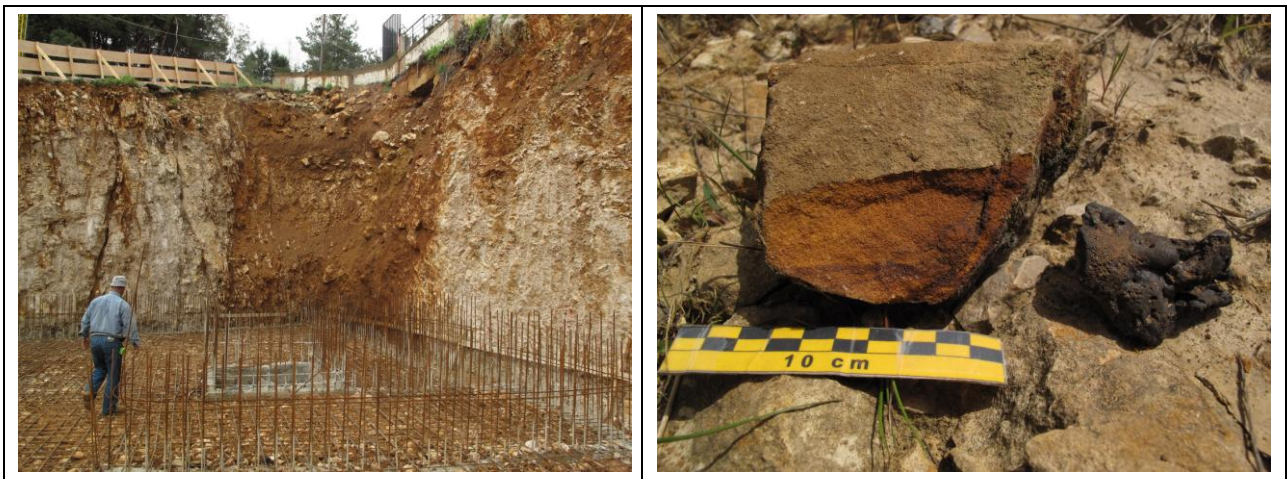
Figure 6: Left: View along strike of a vertical fault trace in Kesrouane Formation (J4) filled with limestone breccia (WP 412). Right: Ferruginous sandstone and iron concretion of a fault with former hydrothermal activity due to widespread basaltic intrusions (WP 038)
