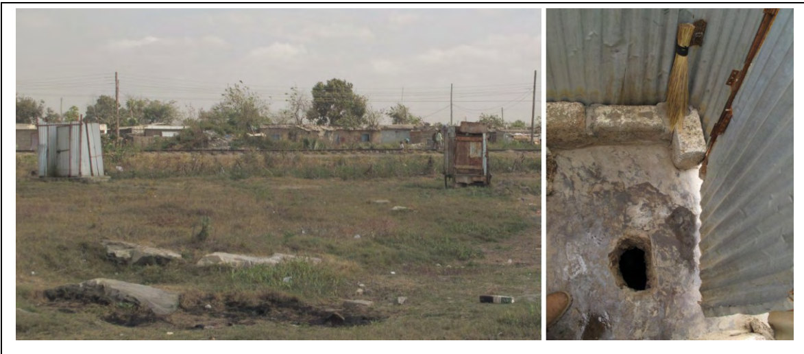
Figure 63: Pit latrines discharging directly into karst holes (WP 016).
