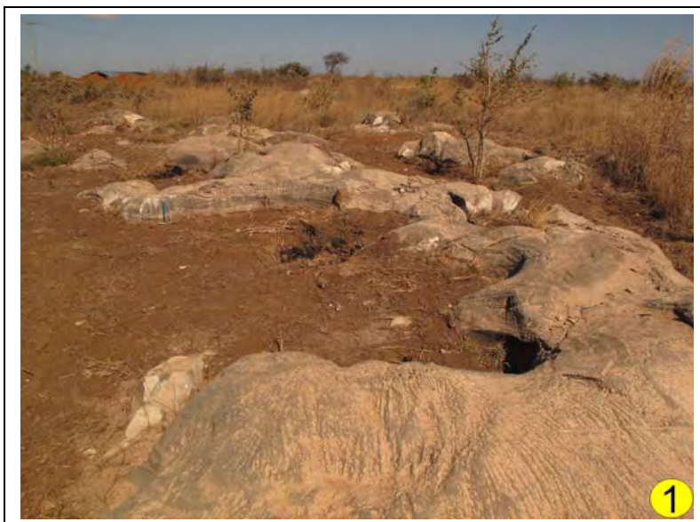
Figure 46: Large soil-filled karst holes in development area. View to 170° (WP 111).
