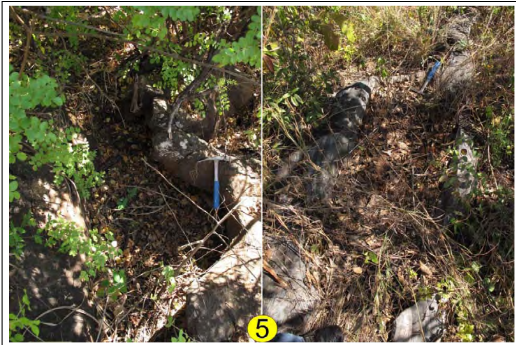
Figure 43: Soil-filled karst holes (WP 043).
