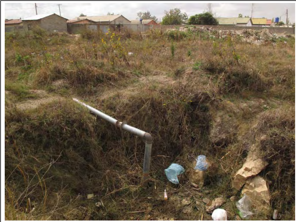
Figure 62: Local water supply of a compound may be affected by ground water contamination from dumping and pit latrines nearby (WP 013).
