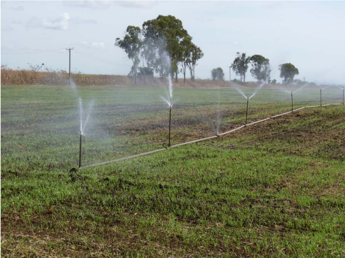
Figure 12: Fixed sprinkler irrigation systems in the project area
