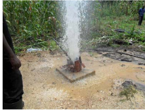
Figure 21: P2/2: Re-development with an air-line
