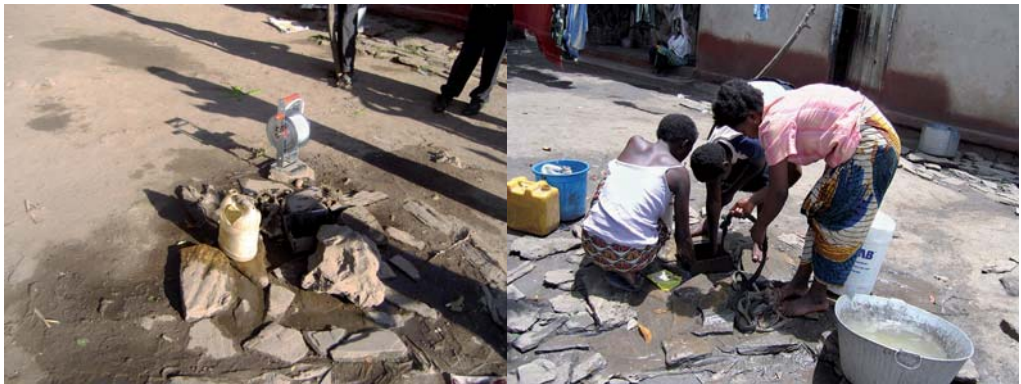
Unprotected shallow wells. Left: shallow well prone to contamination due to run-off. Right: shallow well as source of drinking water.
