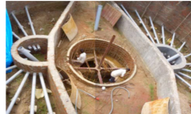
Biogas plant during construction
