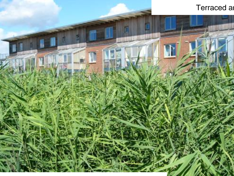
Constructed wetlands (for greywater treatment)
