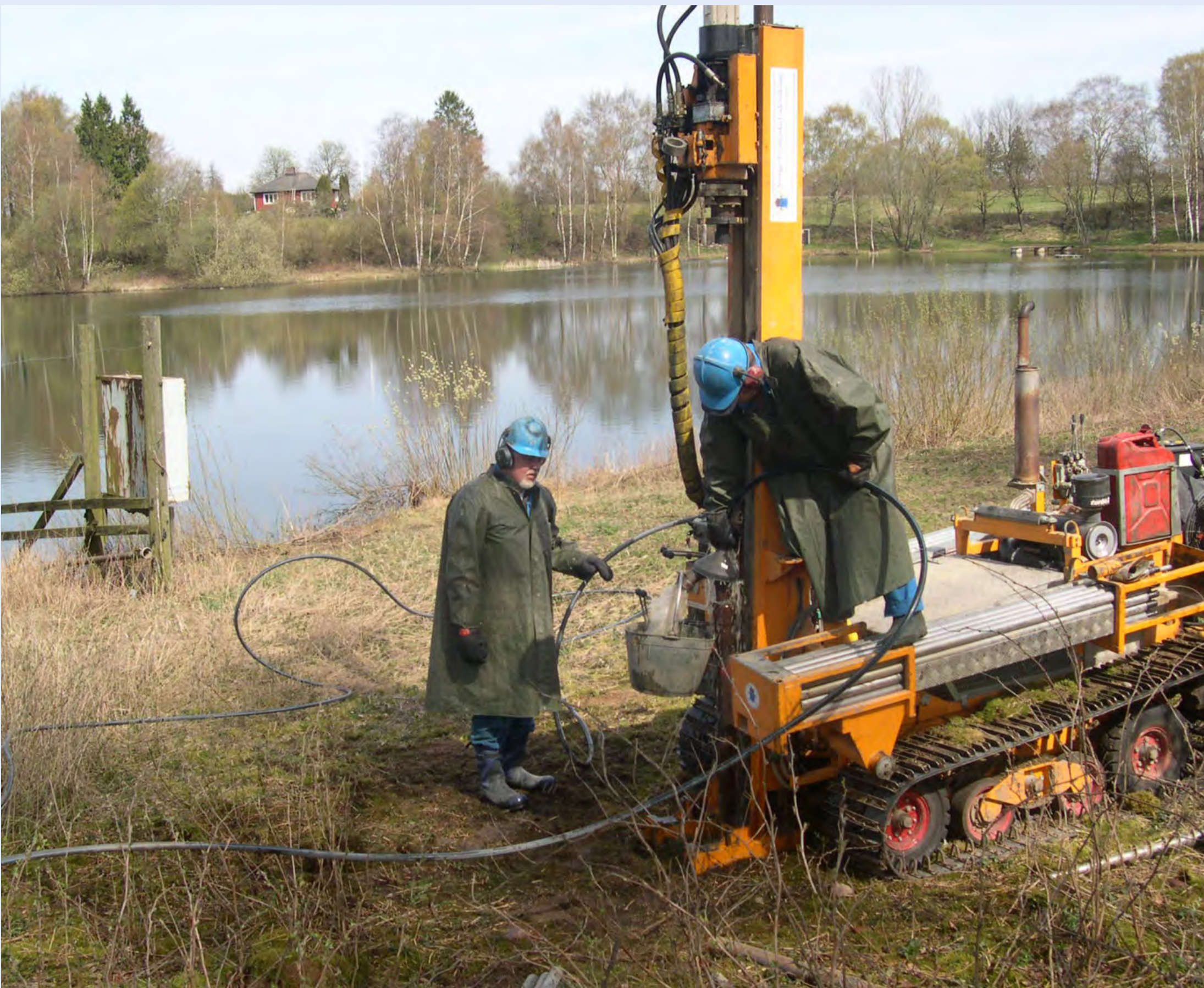
Flushing of groundwater borehole at Bonarpssjön, Ljungbyhed. Photo: Mattias Gustafsson.
