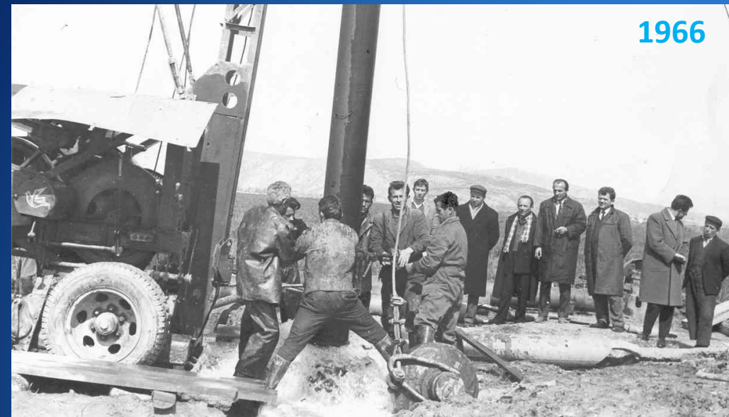
The construction of an artesian well free flowing about 100 l/s in Fushe Kuqe alluvial basin; the authorities are satisfied ...
